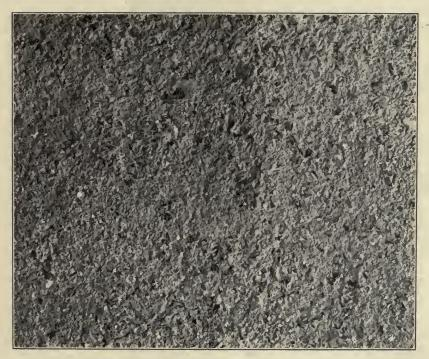
FIG. 8. SAND BLAST TREATMENT OF CONCRETE SURFACE.
