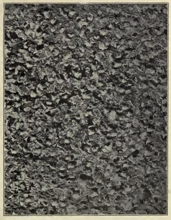
FIG. 10. SURFACE FINISHED BY PNEUMATIC HAMMER.
