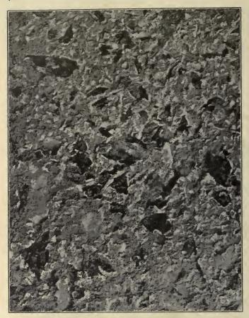
FIG. 9. SURFACE FINISHED BY HAND HAMMER OR AXE.
